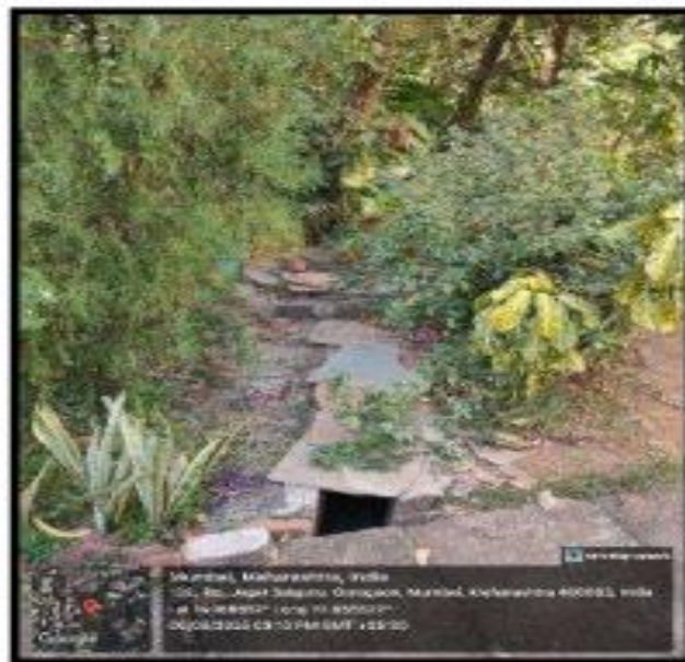
Rain Water Harvesting in Extension Centre
