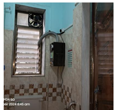
Handle access and Disabled friendly rest rooms
