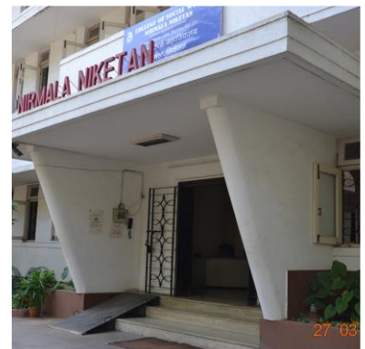
Wheel chair Access Ramp
