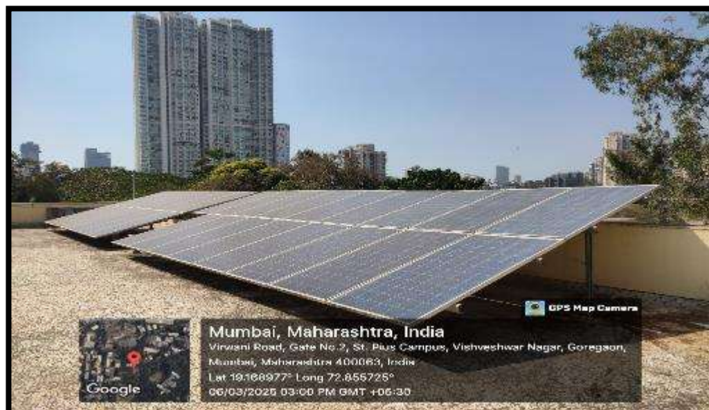
30kW Solar PV System Installation on Extension Centre Rooftop
