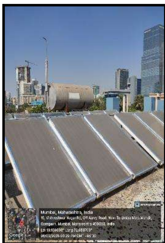
Solar Water Heater Installation In Extension Centre
