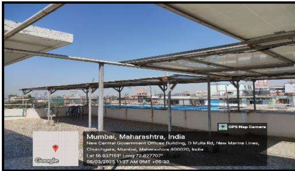
10kW Solar PV System Installation on College Rooftop
