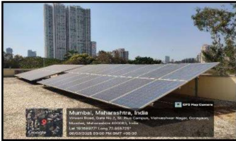
30kW Solar PV System Installation on Extension Centre Rooftop
