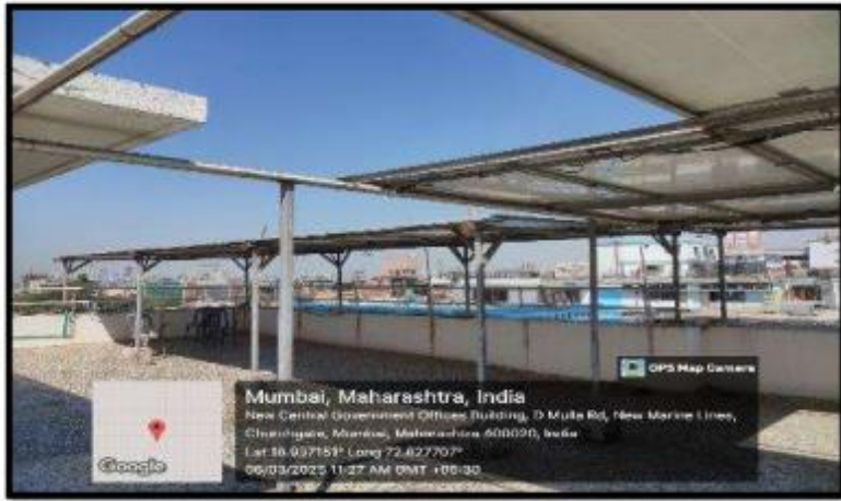
10kW Solar PV System Installation on College Rooftop
